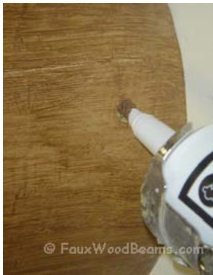
12. Put caulking over the screw heads to hide the screws.
