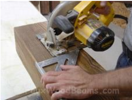
10. Measure length of support structure at the bottom to determine beam length. Cut beam to overall desired length.
