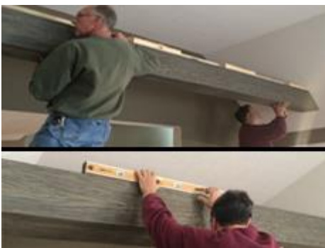
13. Raising The Beam Raise beam onto support structure. Check that both ends are flush with ceiling and beam is level.
