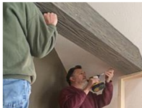
14. Secure beam by screwing into support.
