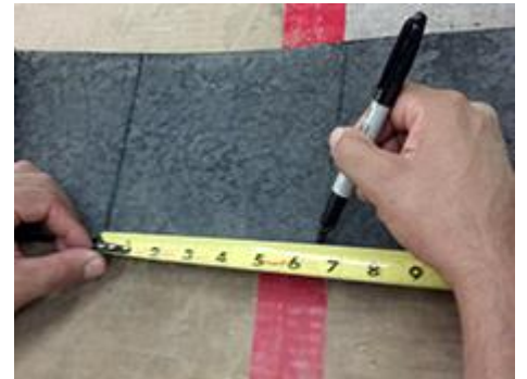
3.) Draw one line on either side of the center line. The new lines should be half the beam's width + 3/8 inch.
