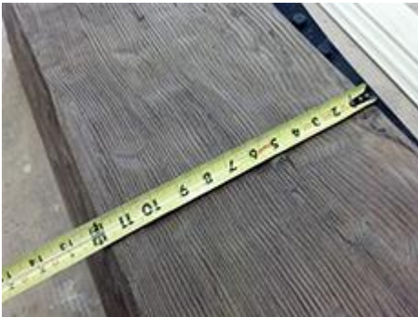
1.) Measure the width of the beam.
