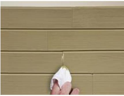
10.) Use a damp cloth to remove any excess textured caulk before it dries. A wet finger, paint brush, or other similar tool can assist in smoothing and blending the caulk. Also use the textured caulk to fill in any voids, gaps, screw heads, or spaces.
