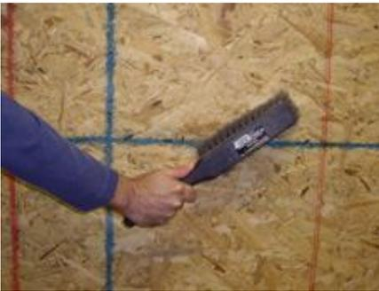
1.) Begin your exterior design project by first by making sure that the wall you're attaching the faux wood to is clean. Wipe down the surface and use a wire brush on harder surfaces. Wipe the back of the faux wood panel as well.
