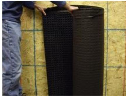
2.) This step shows how to use a drainage mat behind the panels in your exterior design. Roll out and apply the faux panel Drainage Mat to the entire exterior wall to be covered. Use the adhesive/glue behind the mat and exterior-grade staples through the mat into the wall to firmly attach the mat to the wall.
