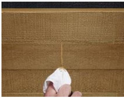
11.) Use a damp cloth to wipe off any excess textured caulk before it dries. A wet finger, paint brush, or other such tool can assist in smoothing and blending the caulk. Use the textured caulk to also fill in any voids, gaps, screw heads, or spaces.
