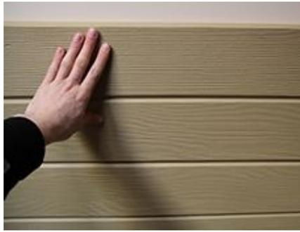
5.) Apply the faux panel to the wall. Use a slight twisting motion to ensure good contact between the adhesive/glue and the wall for proper panel installation. Make sure the panel is level.
