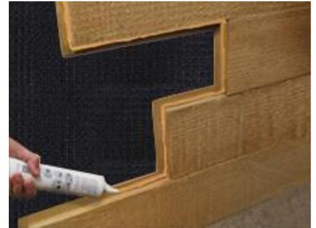
9.) Add the textured caulk to the crease where the panels will meet. This is very important to ensure a weather-tight seal.
