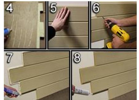
9.) Repeat steps 4-8 for the next faux panel to be installed. Place it onto the wall next to the first panel. Keep the panel level. Press the panels tightly against the wall with a slight wiggle motion to help spread the glue for a tight seal.
