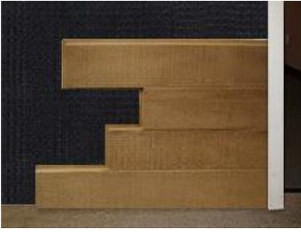
4.) Cut into the first panel by either 1/2, 1/3, or 1/4 and not just cut off the tabs at the end. This reduces the amount of waste, ensures that the seams on the next rows will not line up and will make the install look more realistic.
