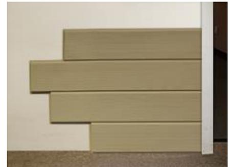
3.) Cut into the first panel by either 1/2, 1/3, or 1/4 and not just cut off the tabs at the end. This reduces the amount of waste, ensures that the seams on the next rows will not line up and will make the install look more realistic.
