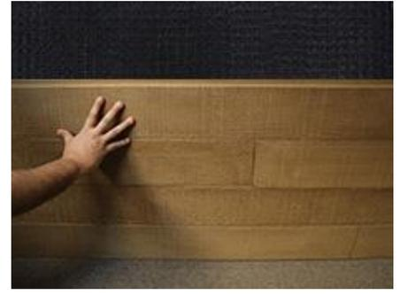
6.) Apply the faux wood panel to the wall. Use a slight twisting motion to ensure good contact with the glue/adhesive and the wall. Make sure the panel is level.
