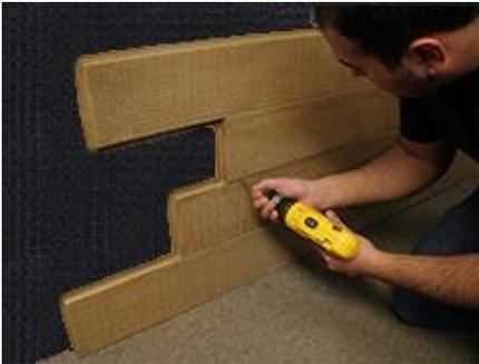
7.) Begin fastening the faux wood panel to the outside wall with screws all around the perimeter at roughly one foot apart or less. Additional screws should be placed in the middle of the panel at a rate of about 1 screw per square foot. All screws should be very slightly recessed below the surface of the panel. Do not over tighten the screws.
