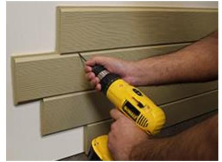
6.) Fasten the faux wood face panel to the wall with screws around the perimeter, keeping them roughly one foot apart or less. Place additional screws in the middle of the panel at a rate of about 1 screw per square foot. All screws should be very slightly recessed below the surface of the faux wood faux panel. Do not over tighten the screws.
